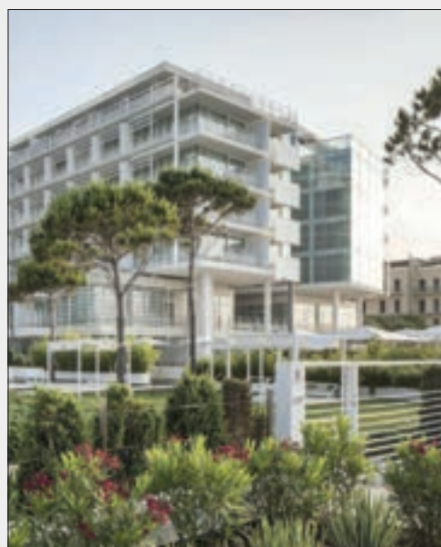
PROJECT MANAGEMENT 5* FALKENSTEINER HOTEL, JESOLO
